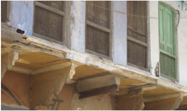
Fig. 3 : Traditional Architecture of the city of Madanganj *
